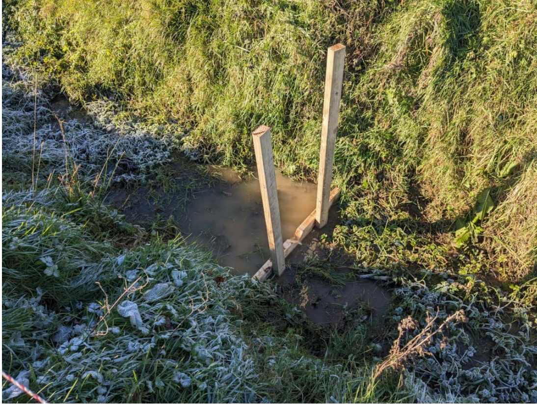
Leaky Dams in open drain (ditch)
